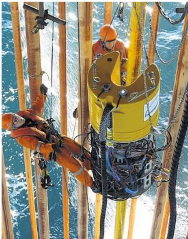
**MEC-Hug Crawler being deployed onto flexible risers**
