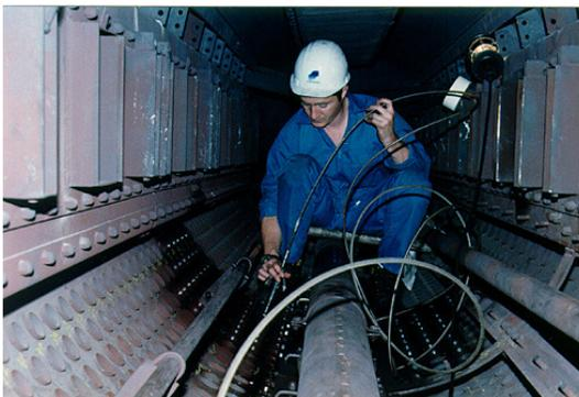
Inspection of steam drum. Tubes are plugged from the mud drum and filled with water
