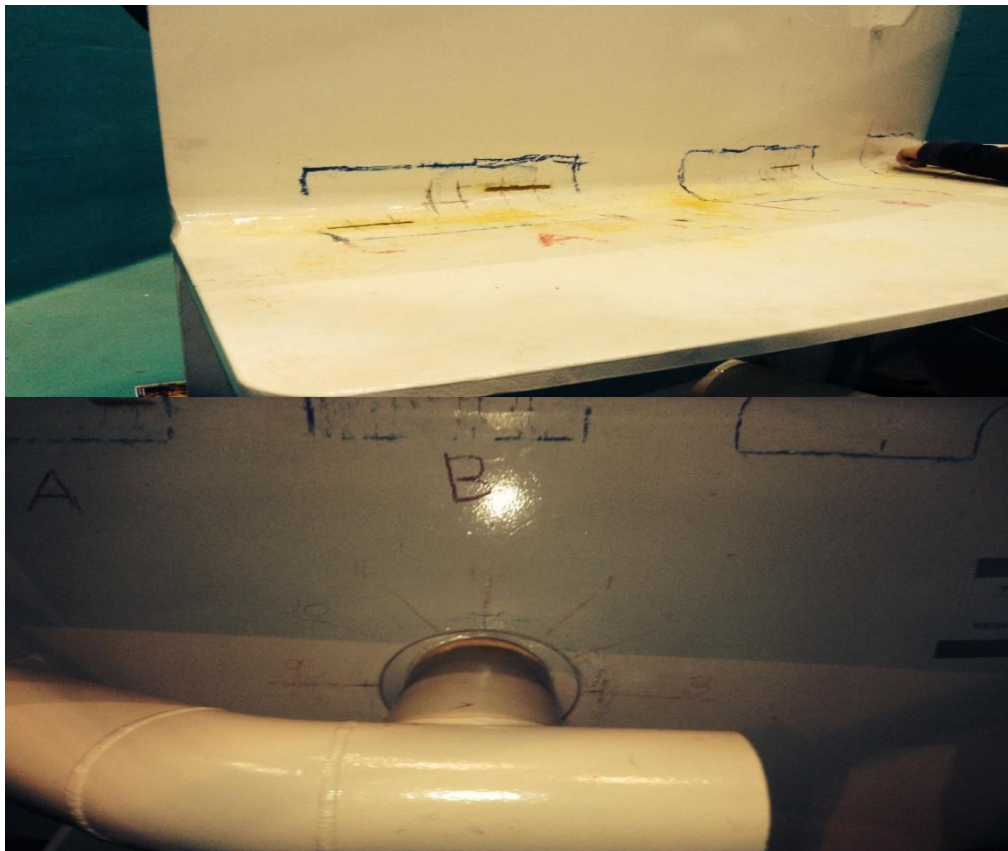
Picture 9 and 10: Showing inspected area locations.
